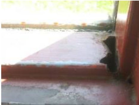
Metal Window Frame
